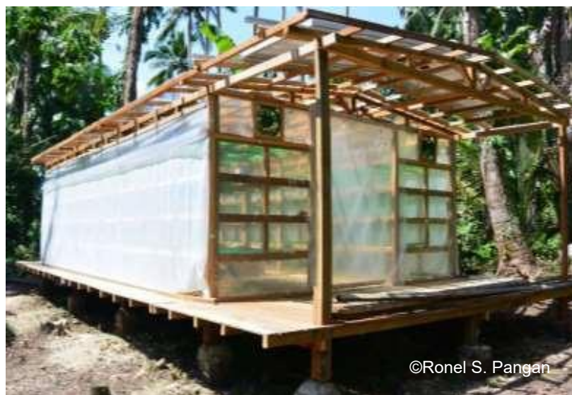
Figure 1. The permanent-type seaweed dryer constructed in Perez, Quezon.
