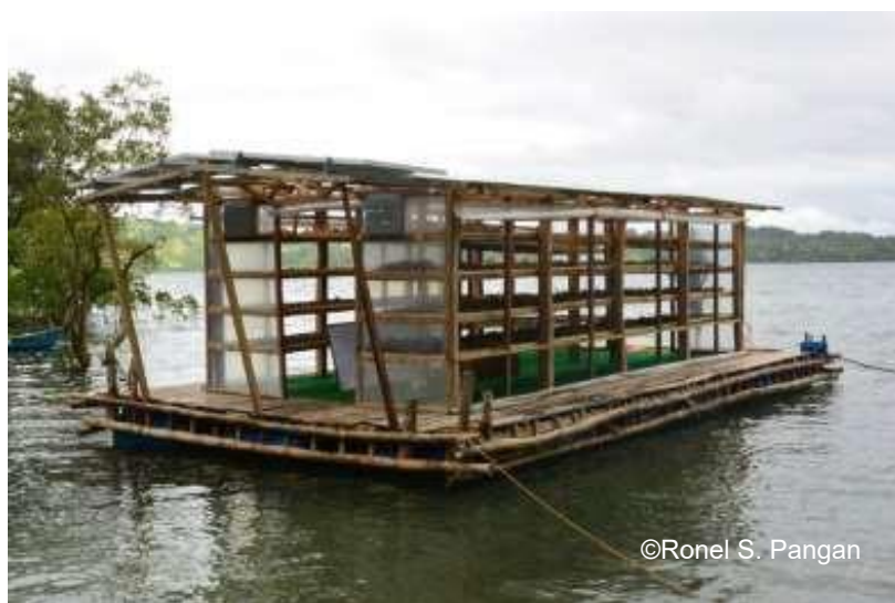
Figure 2. The floating-type seaweed dryer constructed in Looc, Romblon.
