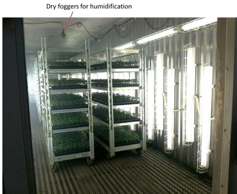
Figure 6. A healing facility developed in a commercial grafting nursery, with lamps protected with water-proof sleeves. (Photo by Chieri Kubota)
