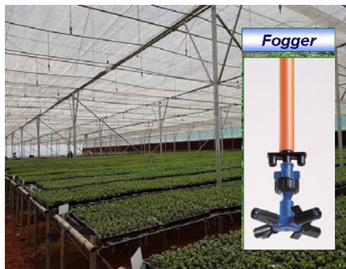
Figure 12: Fogger installation in a nursery
