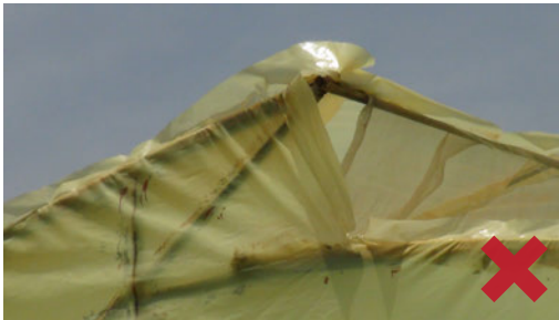
Ensure no gaps in the polythene cover
