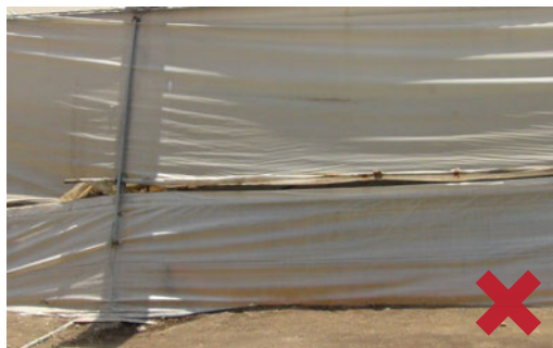
Do not leave gaps in the structure
