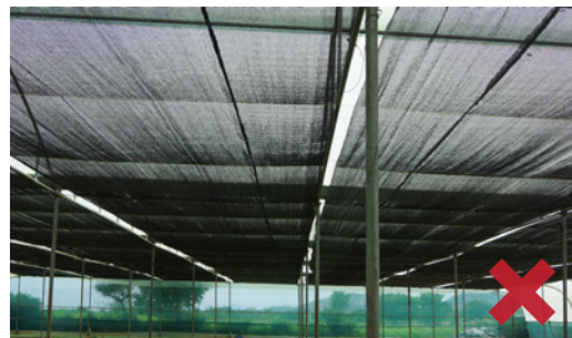
Avoid black shade net under the roof during winter months
