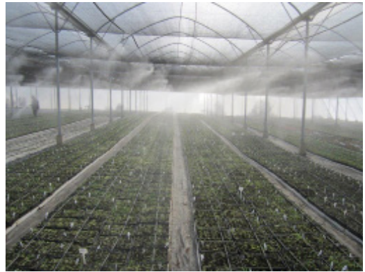
Figure 13: Functioning of foggers triggered by sensors
