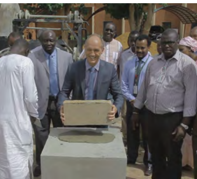
Marco Wopereis sets the keystone for the Center's new two-storey office and lab building at Samanko Station, Bamako, Mali.
