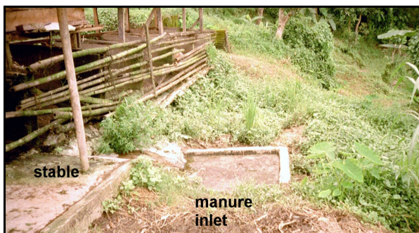
Photo 5.45: Placement of inlet below the stable, Kalimpong subdivision
